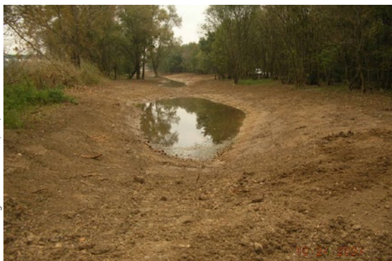
Earthwork to restore a side channel and ponds. October 2007.
